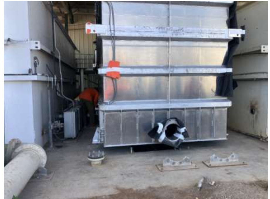
Delivery and placing filter unit in position February 3, 2025
