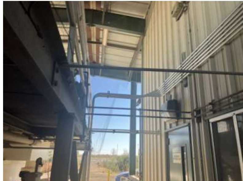
Filter in place; electrical conduit from new filter unit to control room
